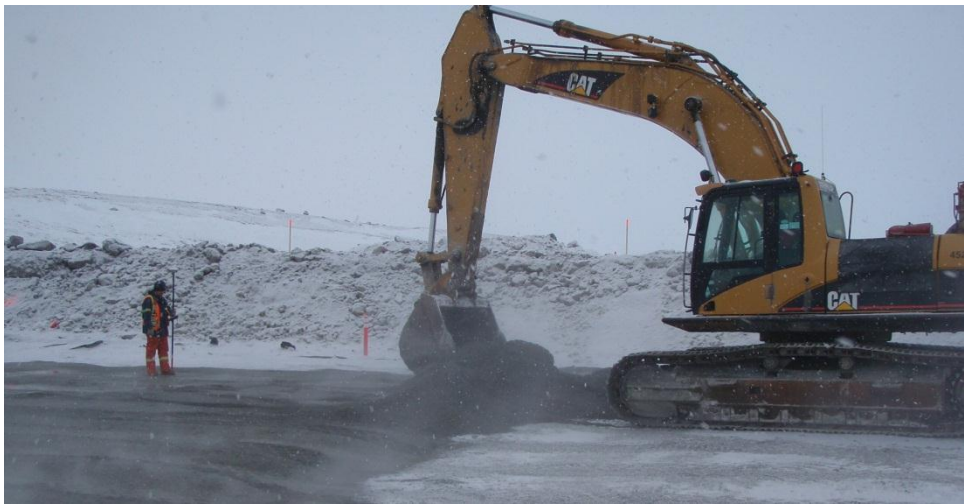
Photo 3: Survey working with excavator to ensure placement is at or below liner grade.
