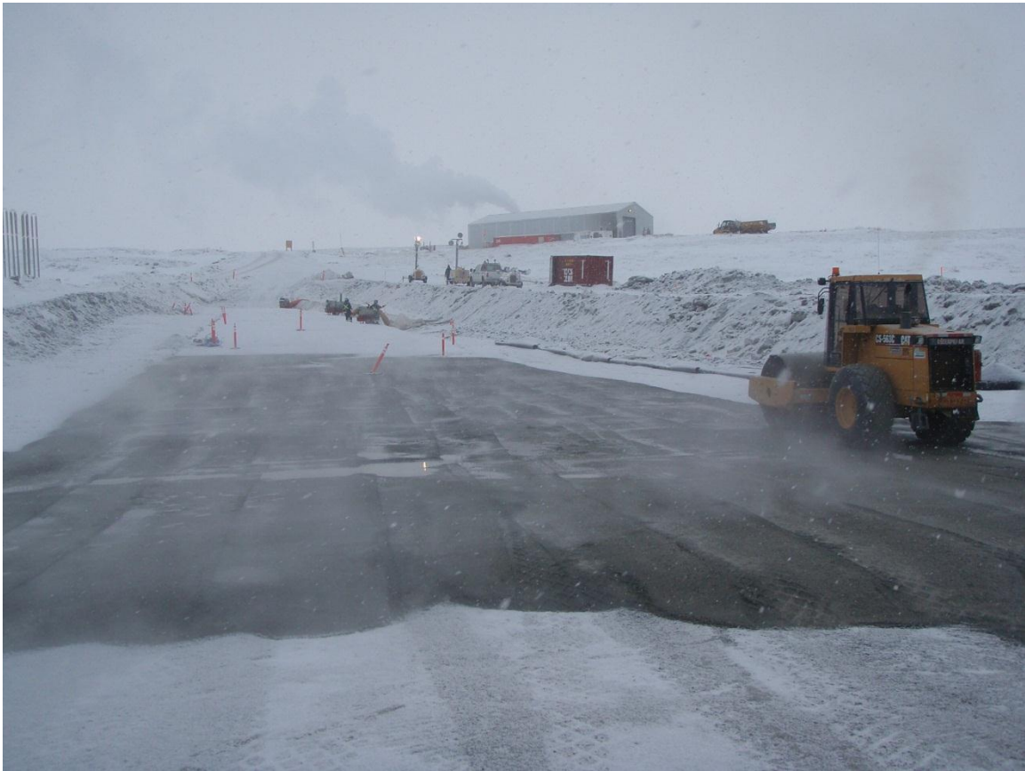
Photo 5: FCM placement. Some water bled out of the material over time.
