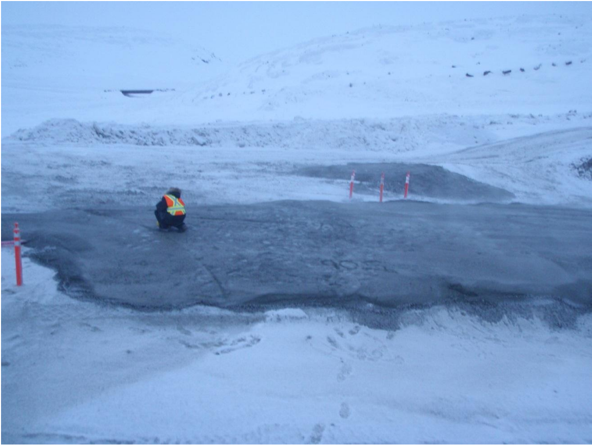
Photo 6: Placement near the south end of the dam. Compaction results were slightly (1%) low in one localized area.
