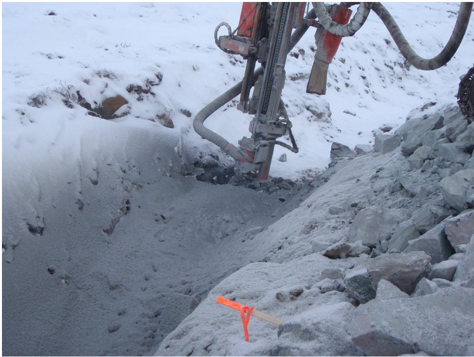
Photo 10: Chipping to obtain grade at the Doris North Diversion Berm.
