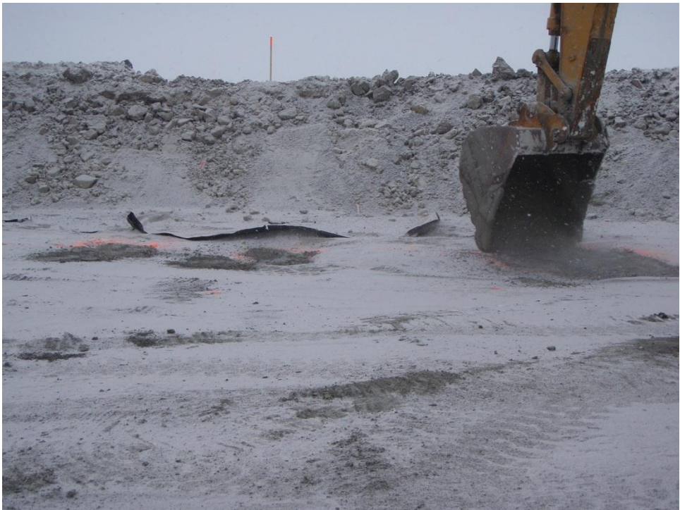
Photo 3: Cat 330 excavator scratching areas of frozen 5/8 clear to be removed prior to placement.
