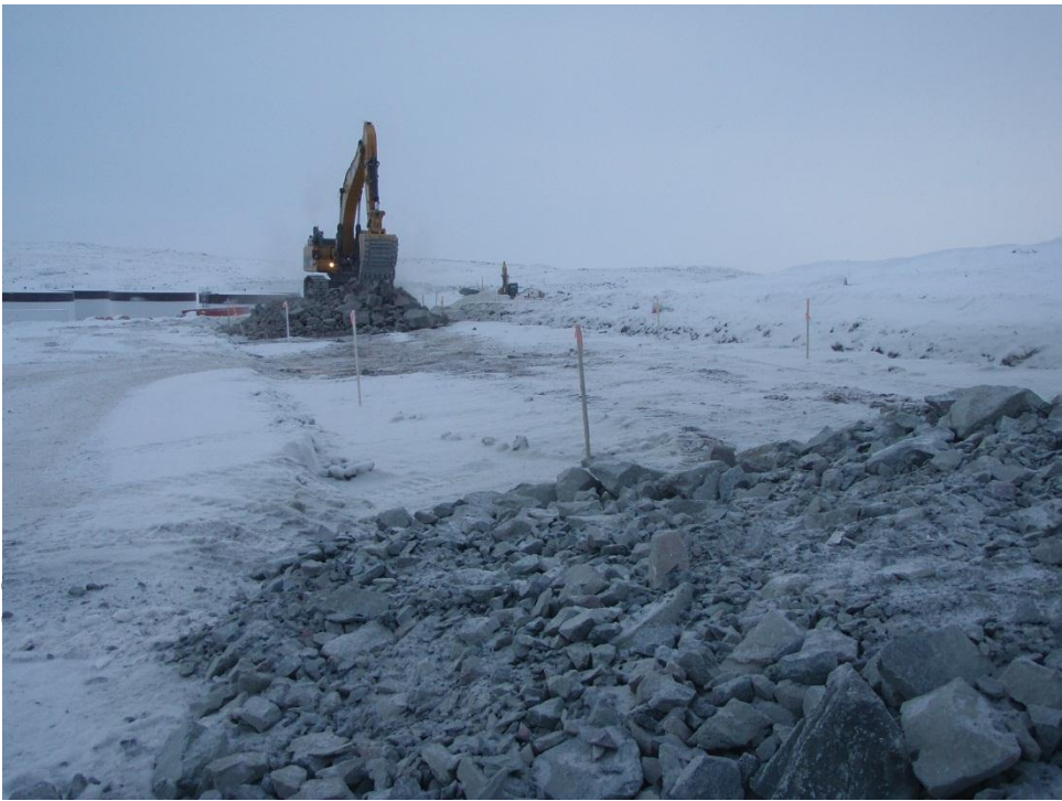
Photo 13: ROQ placement at the Doris North Diversion Berm.
